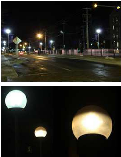
Figure 10. Upper Panel: Unshielded “globe” lights galore on Franklin Street. One of the student dorm buildings can be seen toward the right of the image. Lower Panel: An example of an unshielded light fixture (“globe lights”) housing a T = 5000 K (blue/white color) light bulb and another fixture fitted with a “dark sky reflector” housing a T = 3000 K (off-white) light bulb. T \leq 3000 K light is known to cause less glare and is less detrimental to the environment and plant and animal health (Intl. Dark Sky Assoc. 2010; Luginbuhl et al. 2010).
